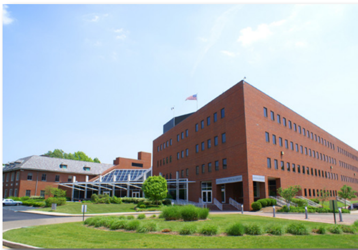
IMG World Headquarters, Indianapolis, Indiana
